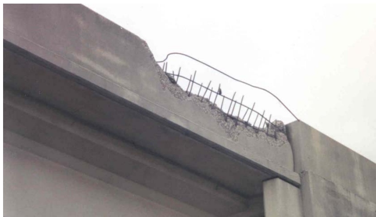
Figure 29. Damage to a 32" concrete bridge railing in a crash with a single unit truck in Florida. [Alberson04]
